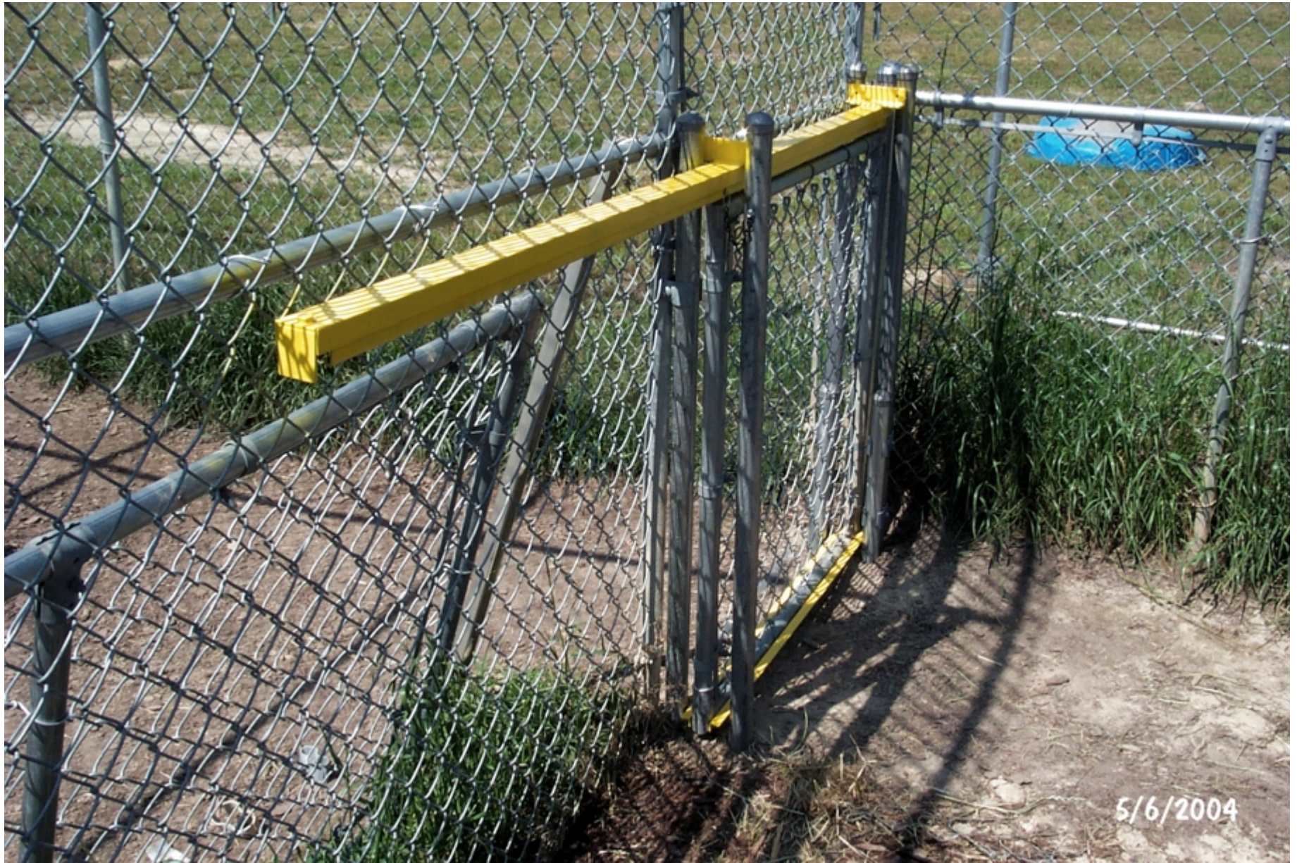
Slide door between wolf cages. Field constructed door (schedule 40 galvanized poles and chain link) was used with our top rail and bottom guides. The top rail has a simpler 90 degree angle steel setup that's screwed to the vertical poles. The top rail and roller setup is the same used with the welded doors.
